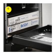
Insert new MERV 11 filter with airflow arrow pointing up.
