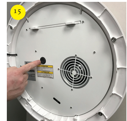
Rubber grommet is now in place.
