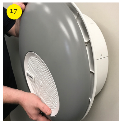
Push front cover back into place.
